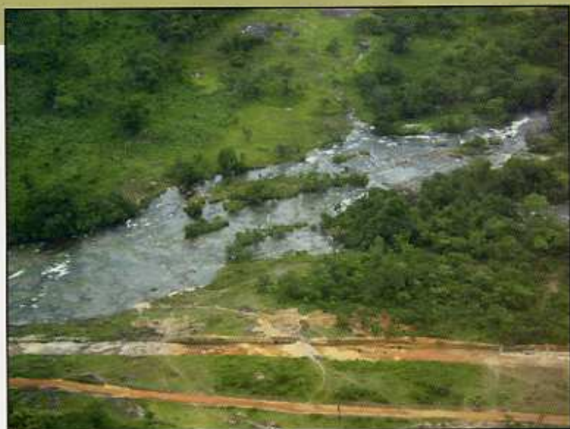
The rapids where the hydro-electric facility is being built.
